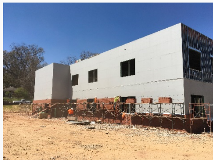
Exterior Framing, Sheathing, Air Barrier, & Brick
