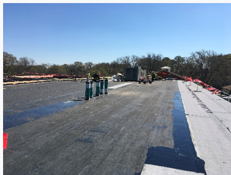
HVAC Units Set & Roofing Installation
