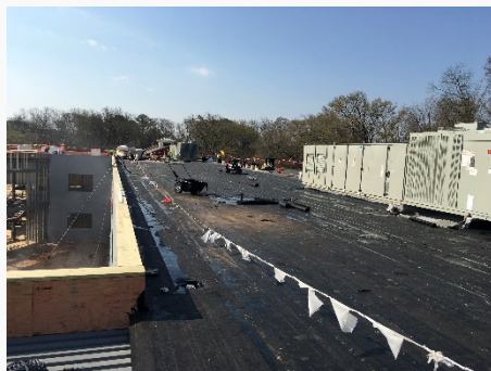
HVAC Units Set & Roofing Installation
