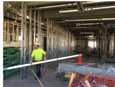
Interior Framing at New Building
