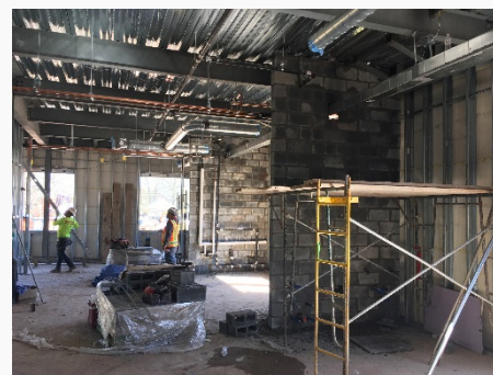
CMU Walls & MEP Installation at New Building
